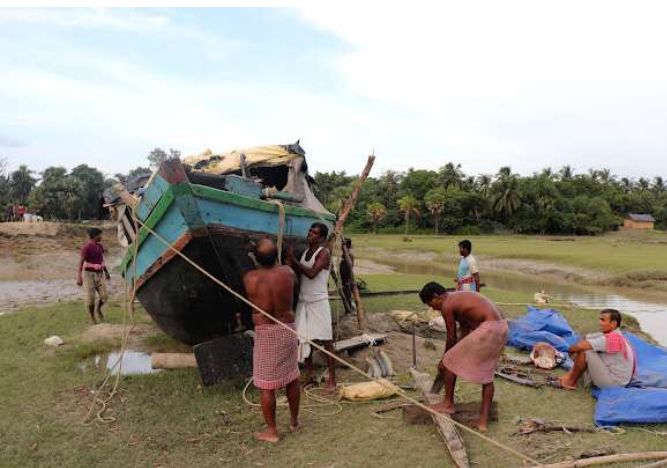
Figure 10 : Repairing of boat takes place after dry docking. Indigenous method of dry-docking where after anchoring to a relatively high land of the bank at the time of high tide and then removing a portion of the clay where it is anchored. Not only boat makers but also family members of boat owners use to take part in the entire process of boat building.
